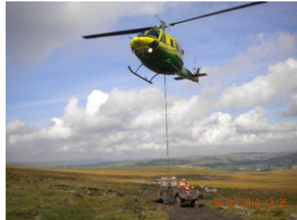
Materials airlifted to site
