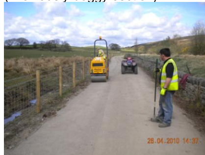
Goit BW during Work (Previously boggy section)
