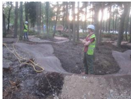
Pump track during construction
