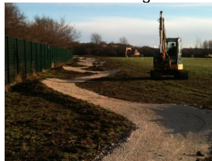
Berm section during work
