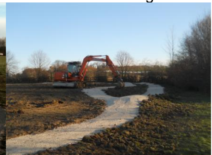
Roller section during work
