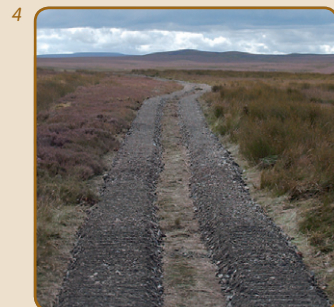
1. Improvement work in progress on an upland public right of way, Darwen, Lancashire; 2. Upland subsoil footpath, Blubberhouses, North Yorkshire; 3. Aggregate track on Darwen Moor, Lancashire; 4. Grass and gravel twin track on the Scargill Estate, Kirkby Stephen, Cumbria.
