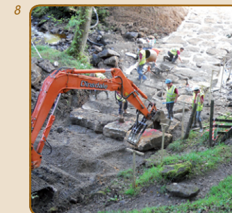
5. Pitched stone track; 6. Single carriage tarmac road at Catlow, Lancashire; 7. Timber built bridge at Ashway Gap, Dovestones Reservoir, Greater Manchester; 8. Ford construction, Thruscross Reservoir, Washburn Valley, North Yorkshire.
