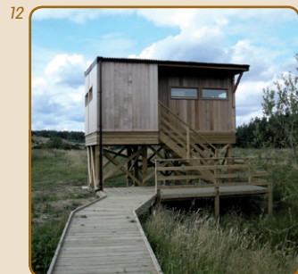
9. Timber gate on the Goit Route, Pennine Bridleway, Chorley, Lancashire; 10. Stone built shooting butt, Caldbergh Moor, North Yorkshire; 11. Footpath and wheelchair access route, National Nature Reserve; 12. Timber boardwalk and bird hide, Foxglove Covert Nature Reserve, Catterick Garrison, North Yorkshire.
