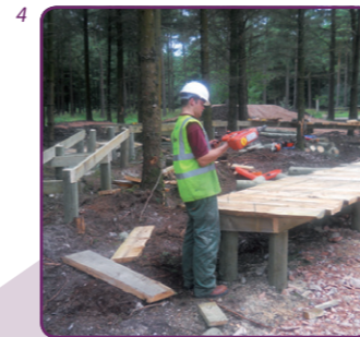
3. Berm construction at a 4 cross track, Afan, South Wales; 4. On-site construction of timber boardwalks in the Skills Area at Haldon Forest Park, Exeter.
